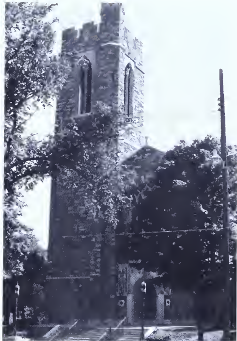
Our Lady of the Blessed Sacrament Church, 2121 North Third Street; mica schist from the Philadelphia area.
